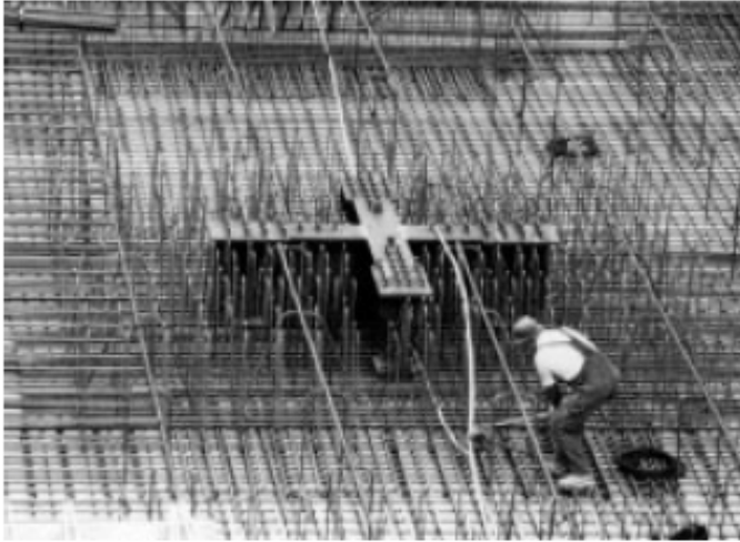
Fig. 9: Steel composite construction for resisting punching shear developed by s+v [22]
