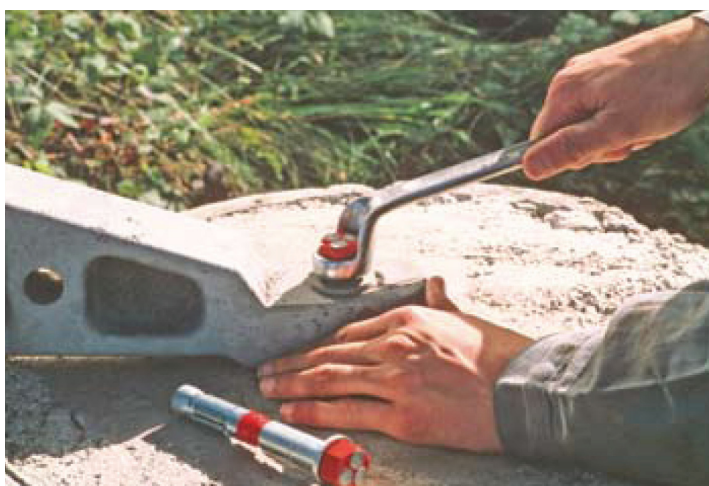
Fig. 2: Torque controlled expansion anchor with red shear-off cap
