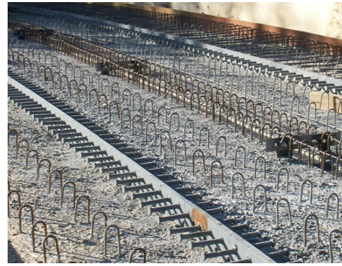
Fig. 17: View on the upper side of prefabricated girders
